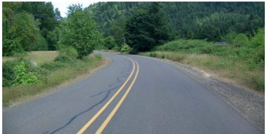
New Asphalt Pavement Overlay
